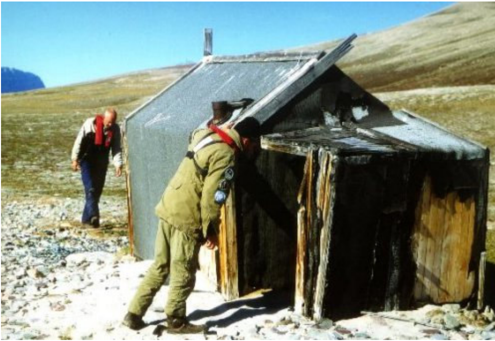
The Kap Ovibos hut before and during restoration.
