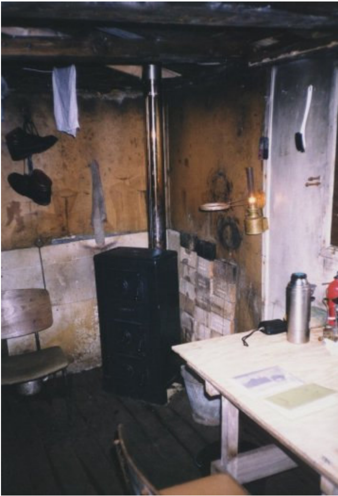
Photo: A new stove has replaced the old, useless one. The oven was put to the test, to dry out the house thoroughly. The old ceiling plates were torn down, so that the beams are not visible. Floor and walls are washed clean of mould and dirt.
