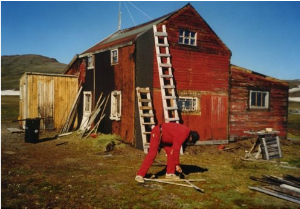
Photo: This is what Myggbukta looked like shortly after arrival. Work has begun. The felt has been removed from the porch. The first lane of roofing felt has been nailed on to the south gable. The roof angle is measured.
