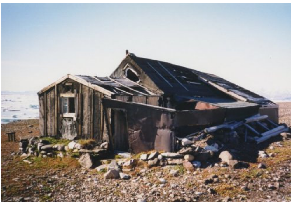
Photo: Cape Herschell station in the summer of 1999. The house in an advanced state of decay, and an expedient restoration is needed if the station is to be preserved.
