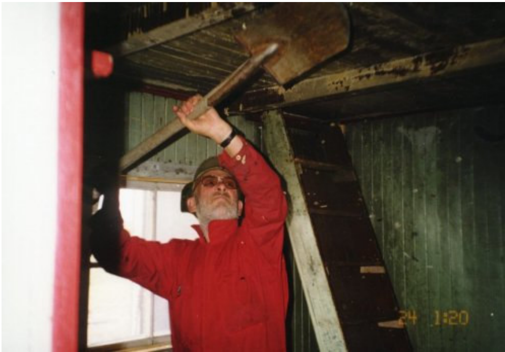
Photo: Øystein cleans the kitchen ceiling of dirt and loose paint.
