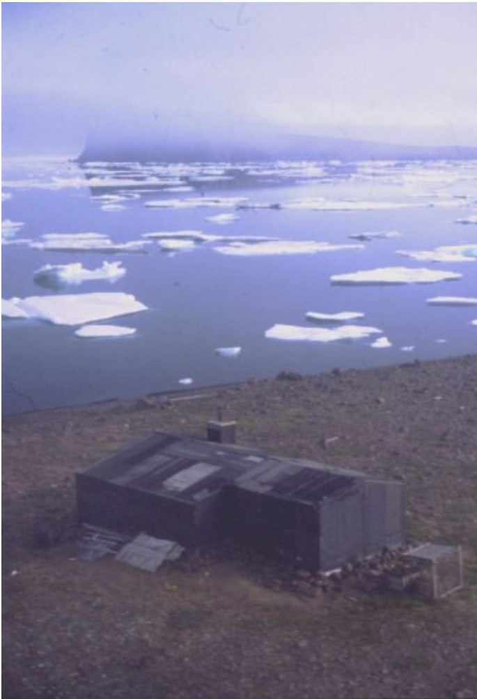
Photo: The helicopter surveillance to Germaniahavn showed that there were large, open holes in the roof. Inside, the walls were running.
