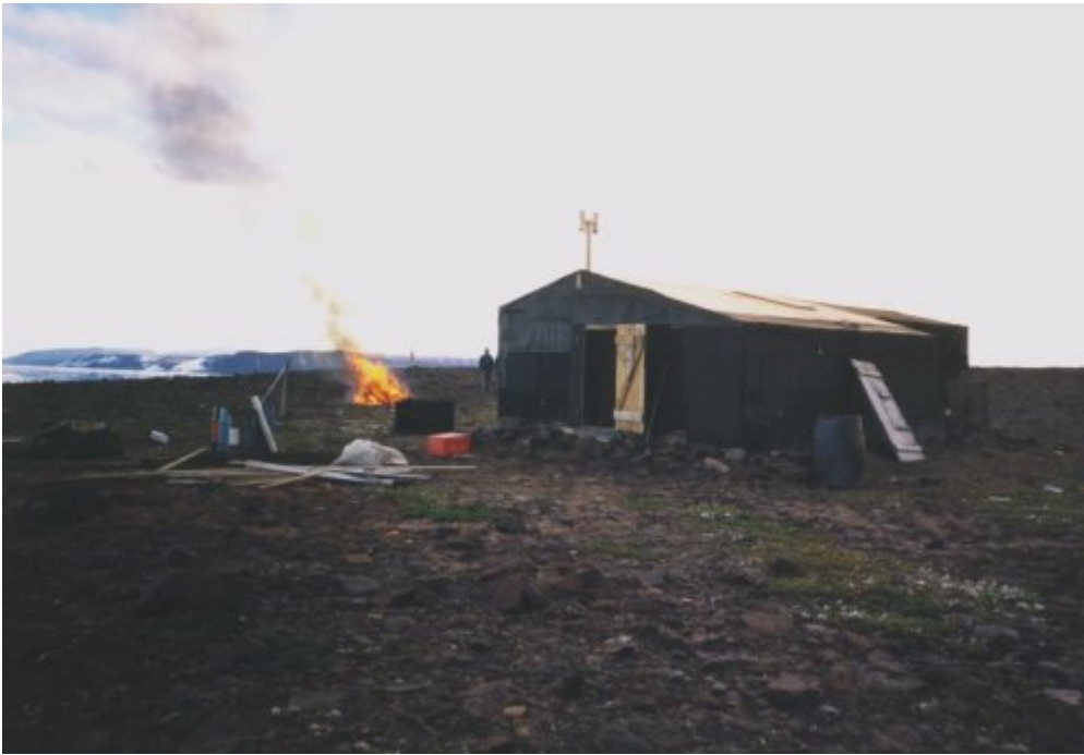
Photo: The old rotten wood from roof and ceiling were burned. The rotten boards were exchanged and the roof waterproofed with plywood plates.
