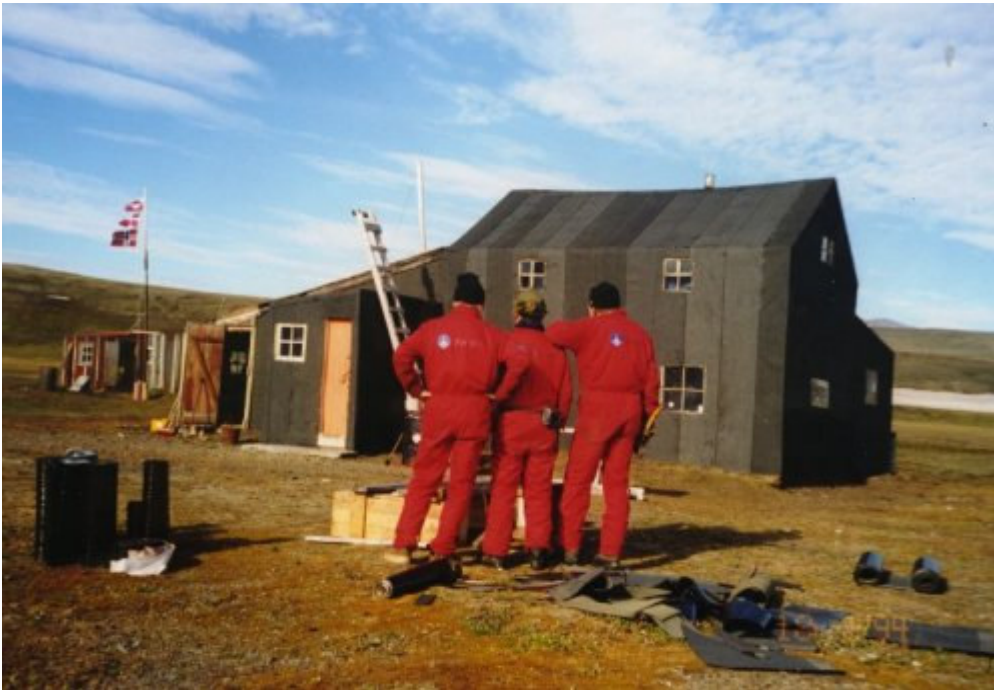
Photo: First phase accomplished. We take a step back to enjoy the sight of the new Myggbukta.
