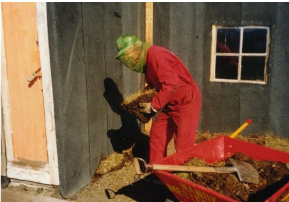
Thor builds a new dirt wall
