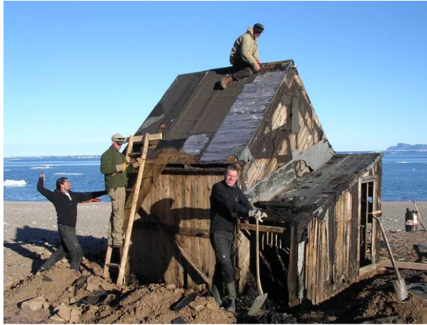
Elvsborg: Start and half way. From the lower edge of the window and up, the major part is original.
