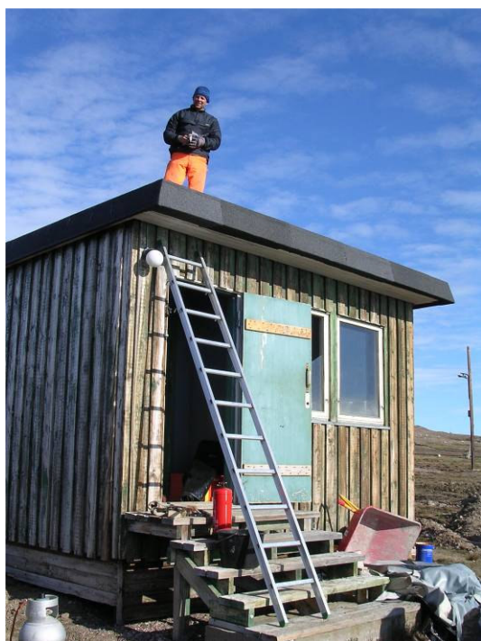
Tagpapterrassen with new roof.
