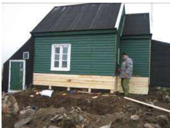
Left: The bottom part of the outer board wall is replaced and reinforced.
