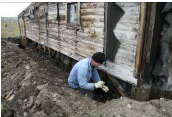
It was necessary to replace the lower part of the woodwork on the rear side of the house due to rot.
