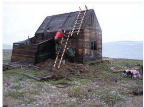
At arrival Laplace was open and moist, but after 12 hours with our mouths full of nails during nonstop work nailing on new felt, the living room was cleared and tight.
