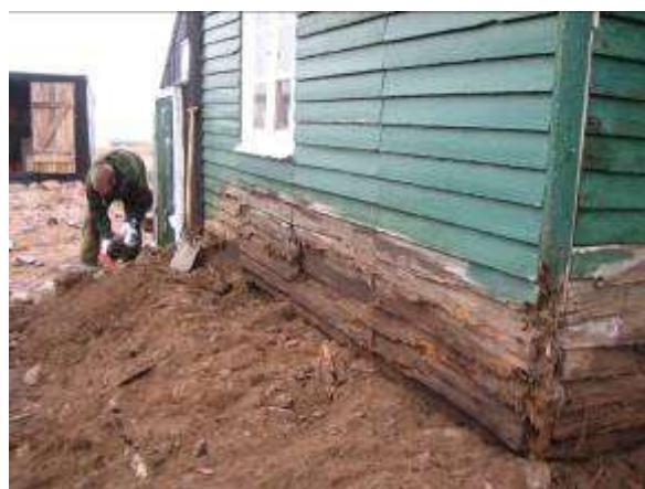
The stone wall in front of the western wall is removed and wet, rotten wall is exposed.
