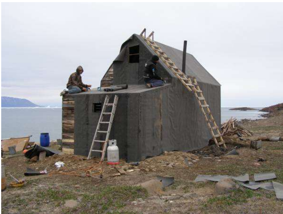
The inner felt is put on, one nail each 10 cm. That sums up to about 10,000 nails!
