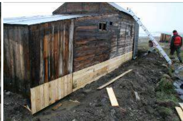
It was necessary to replace the lower part of the woodwork on the rear side of the house due to rot.
