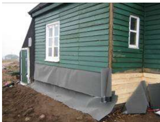
Left: The bottom part of the outer board wall is replaced and reinforced.
