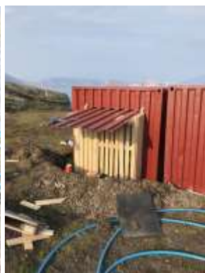
Left: Who needs a fitness centre, when you can dig earth? Middle: Container opened with angle grinder and used as roof for the extension. Right: Extension on the 'boat house'. Newly attached felt, drainage system and grout ought to keep it snow-proof. In addition, weather station with solar cells mounted.
