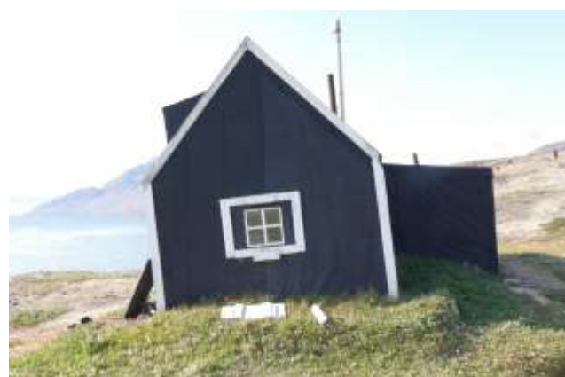
Hoelsbu [356]. The hut is now tilting in such a degree that Nanok is considering a rectification in 2021.
