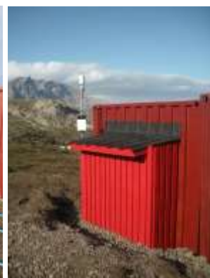
Left: Who needs a fitness centre, when you can dig earth? Middle: Container opened with angle grinder and used as roof for the extension. Right: Extension on the 'boat house'. Newly attached felt, drainage system and grout ought to keep it snow-proof. In addition, weather station with solar cells mounted.
