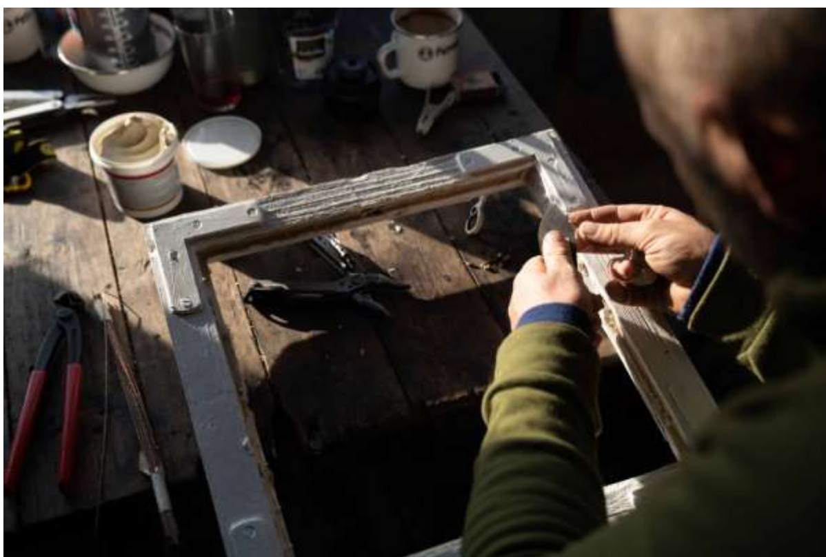
Renovation of Hvalrosodden. Top: Minus degrees and some days with wind and snow. Below: Windows were taken off and repaired.
