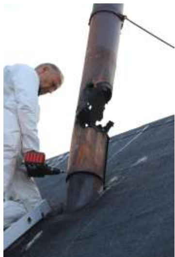
Outdoor renovation. Left: Jesper replacing the corroded stove pipe. Right: The wood was screaming for a new layer of paint.
