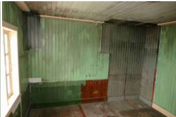
Removal of masonite cladding and stationary cabinets/bunks in the living room. Behind the masonite the fine, old panel walls reappear – with different layers of paint.
