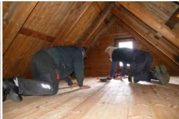
In the attic the old flooring is removed and replaced with an entirely new plank flooring.
