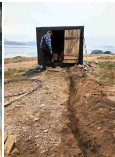
Left: Skindskuret inside upon arrival. Middle: New floor of Skindskuret, and the bed in the new "simple room" is tested. Right: Asger digs down electric cable and ground spear near Skindskuret.
