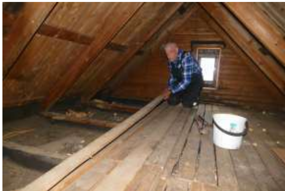
In the attic the old flooring is removed and replaced with an entirely new plank flooring.
