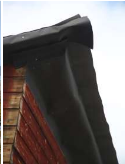
Left: Draining of the surroundings. Right: Weatherproofing of roof against rain and drift snow.
