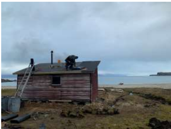
Left: Mounting new roofing felt. Right: New boarding on the back.
