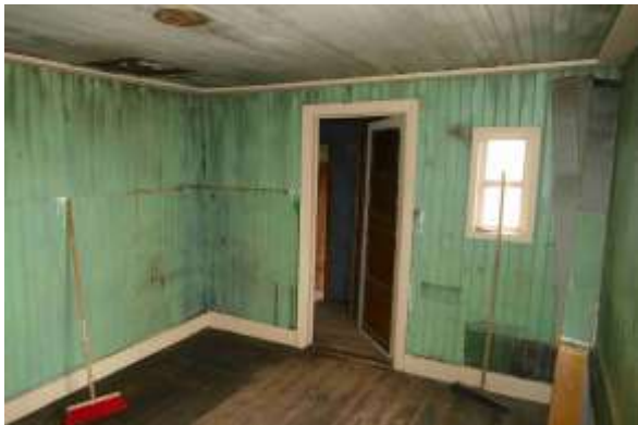
Removal of masonite cladding and stationary cabinets/bunks in the living room. Behind the masonite the fine, old panel walls reappear – with different layers of paint.
