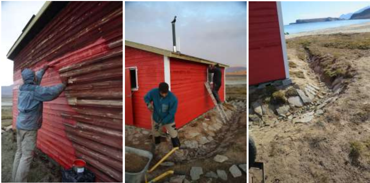
Left: Painting the outer covering. Center: Finishing the ditches. Right: Part of a new drainage.
