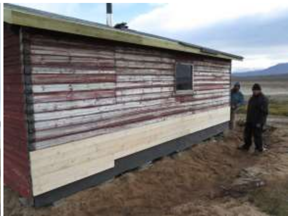
Left: Mounting new roofing felt. Right: New boarding on the back.
