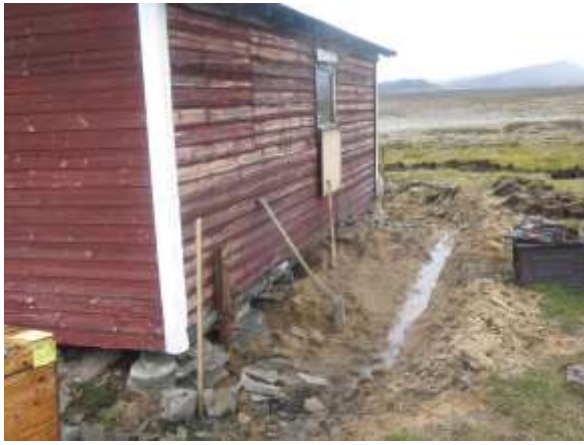
Restoration of Hamna. Left: Draining and laying up. Right: The center of the hut is laid up.
