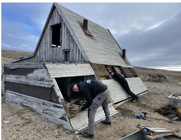
Restoration in process. It was necessary to remove the roof on the eastside of the house to restore the supporting structure.
