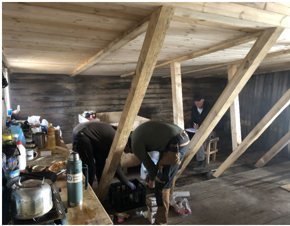
The supporting structure is now restored. Floors and attic will be restored in the next phase - in 2023.
