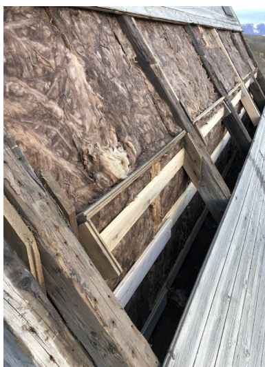
Reparation of the supporting structure of the eastside of the house. Insulation and felting of the roof.
