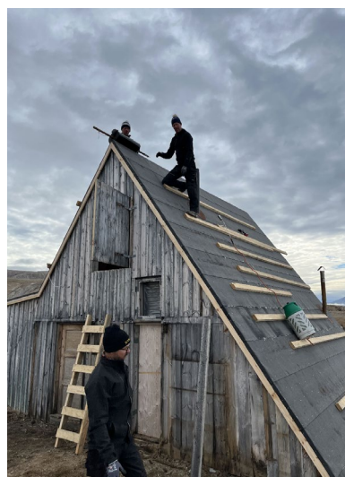
Reparation of the supporting structure of the eastside of the house. Insulation and felting of the roof.
