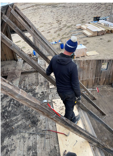
Reparation of the supporting structure of the eastside of the house. Insulation and felting of the roof.
