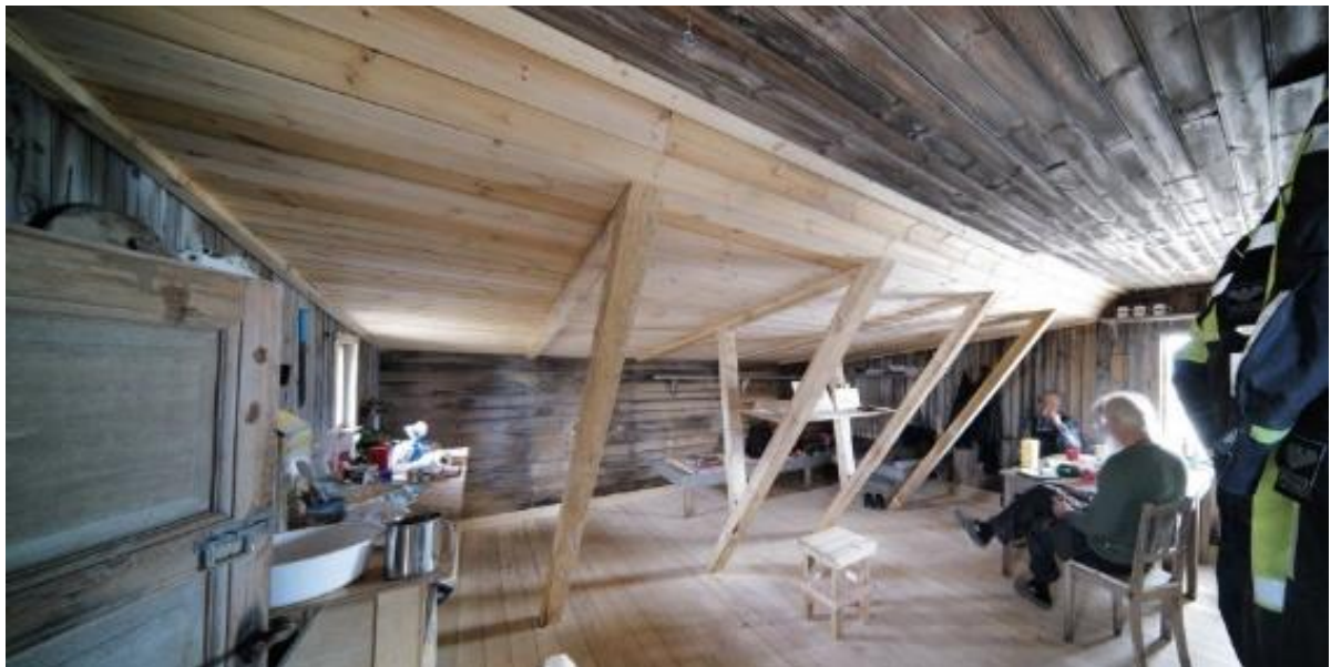
Section of the refurbished large room in Kulhus.
