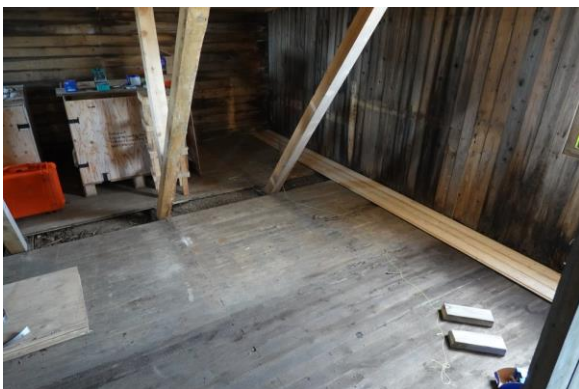
New boards put onto the old floor in the large living room.
