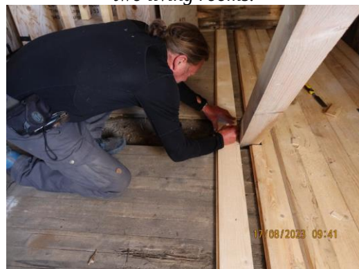
New boards put onto the old floor in the large living room.
