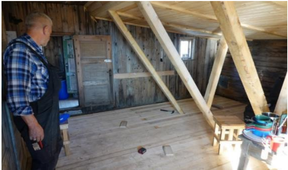
Finished installation of the new floor in the large room.
