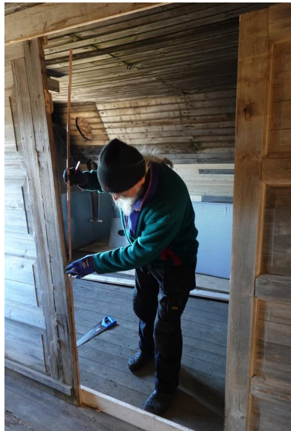
Measuring for installation of door between the two living rooms.
