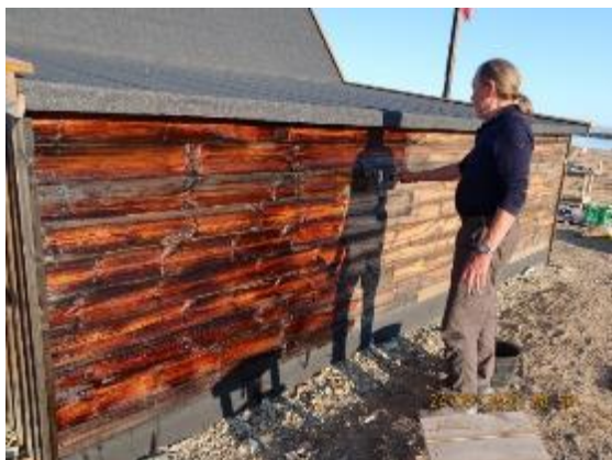
Painting with wood tar – on the extension ...
