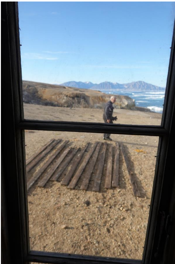
Old floorboards put outside for drying, sorting, and reuse.
