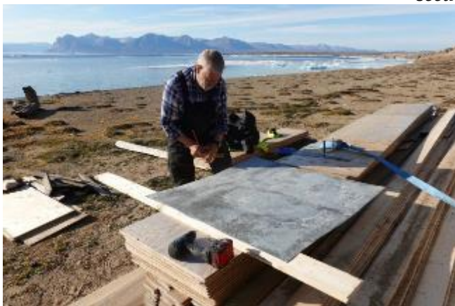
Cutting zinc plate for fire protection.
