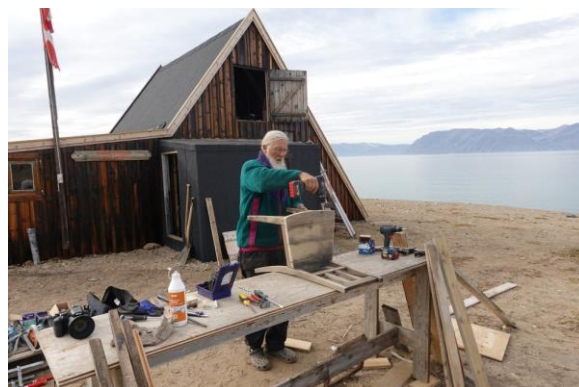
Restoration of old dining room chair.
