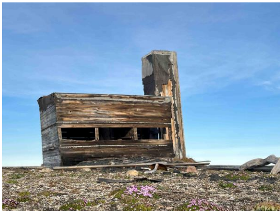
[338] Kap Broer Ruys Nord - or the "Cathedral" as it is also called - is a very atypical cabin with its "church tower". It is not an impossible task to renovate it, but it will require a greater effort.
