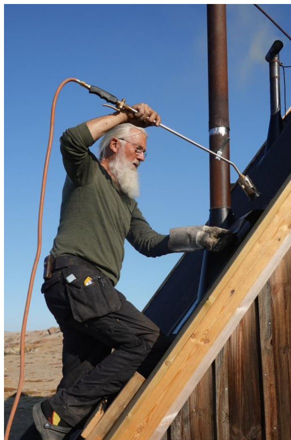
Installation of the stovepipe sealings to ensure that meltwater does not seep through.
