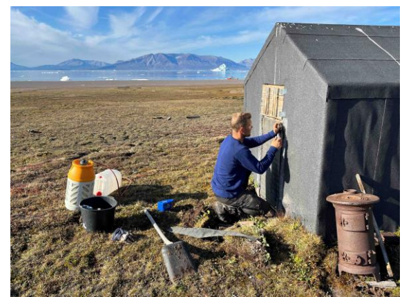
After an exciting renovation task of just over 3 hours, the bear hole was closed, and Smedal was once again ready for guests.
