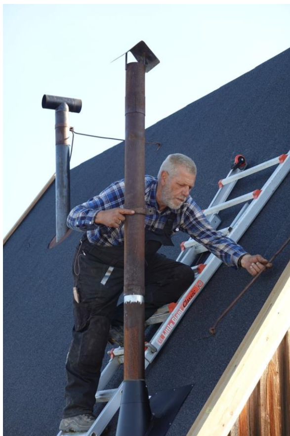
Installation of the stovepipe sealings to ensure that meltwater does not seep through.
