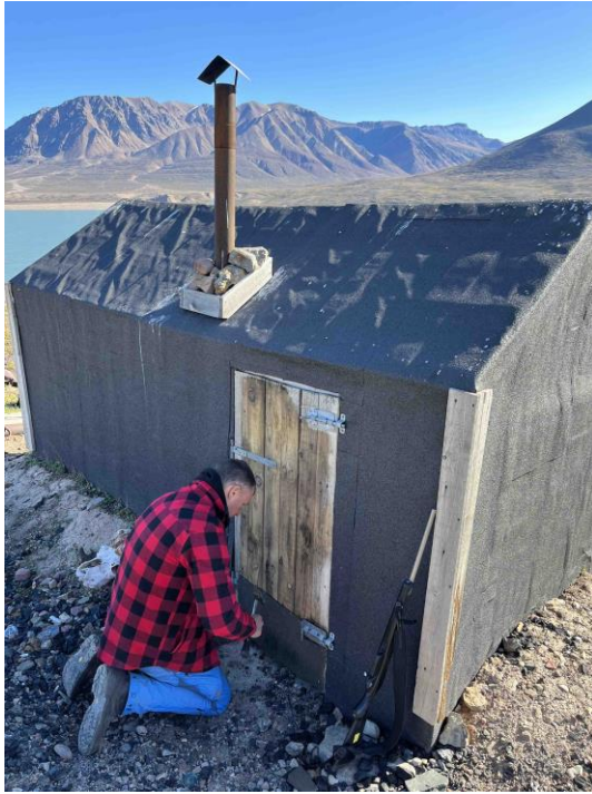
Halle got new roofing felt on the door, and we then continued through Moskusoksefjord.
