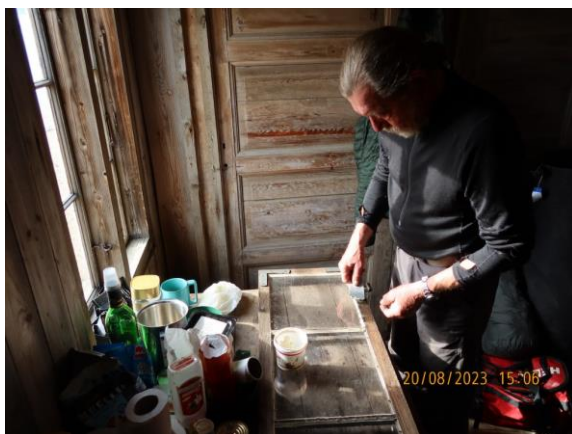
Puttying of the original windows.
