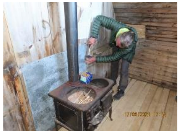
Mounting zinc plate behind coal stove.
