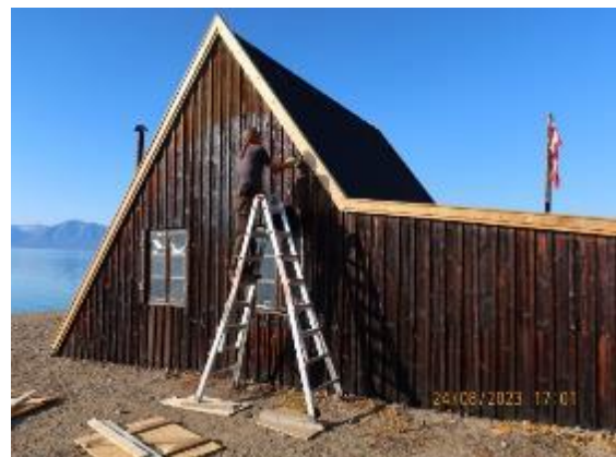
... and on the end of the A-house towards south.
