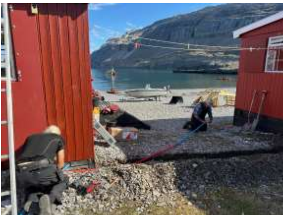
Work on the electrical system at Ella Ø. Leading 230 V into the houses.
