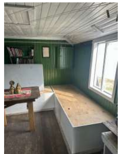
In the bedroom and living room/kitchen, the walls were washed and then painted with green linseed oil paint to match the original color. The ceiling also received a fresh coat of white paint.
