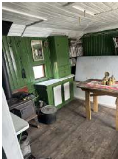
In the bedroom and living room/kitchen, the walls were washed and then painted with green linseed oil paint to match the original color. The ceiling also received a fresh coat of white paint.
