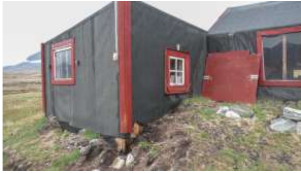
Outside, the foundation was dug free so that new roofing felt could be installed before covering it again.
