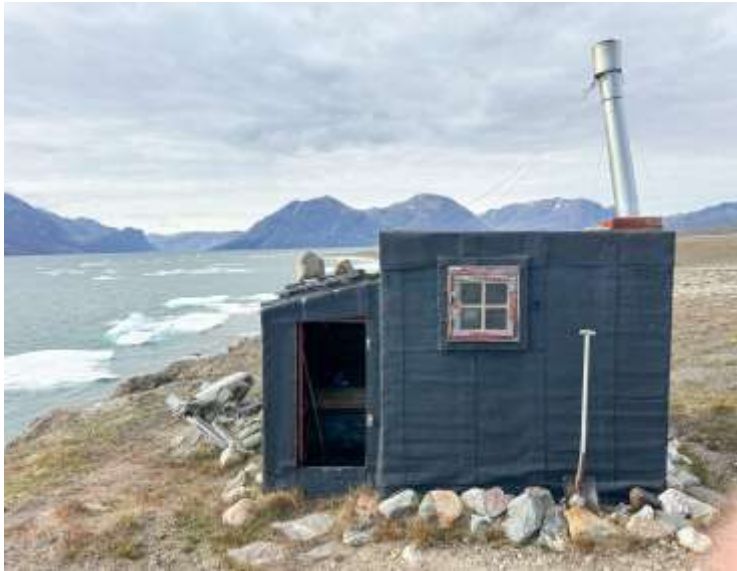
At Pashytten [433], the chimney was secured with wires and straightened.
