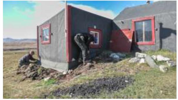
Outside, the foundation was dug free so that new roofing felt could be installed before covering it again.
