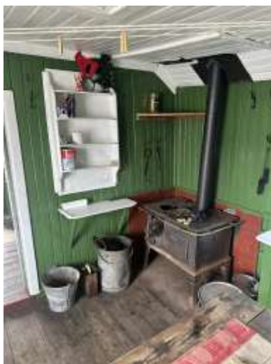
In the bedroom and living room/kitchen, the walls were washed and then painted with green linseed oil paint to match the original color. The ceiling also received a fresh coat of white paint.
