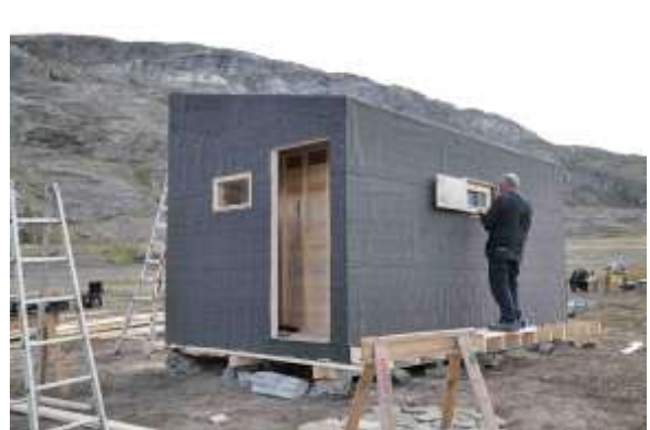
Installation of walls and windows and covering the roof with roofing felt.
