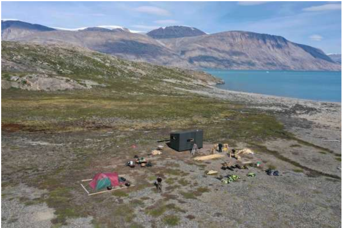
The construction site at Kap Hedlund.
